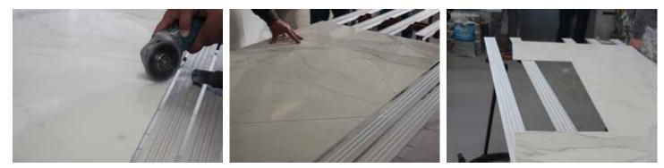
• When manipulating large porcelain panels, a variable speed right angle grinder is strongly suggested to reduce vibration. Electroplated diamond blades or electroplated diamond drill bits should be used for various cuts and manipulations. See page 63-65 for recommended tool providers
