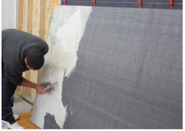
• Large porcelain panels can be installed over concrete or other suitable substrates. You must honor all expansion joints or any defects in the substrate and mitigate prior to installation.
